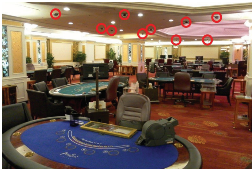
Figure 2.5: Example of large surveillance network in Majestar Casino , Jeju island South Korea [10].
